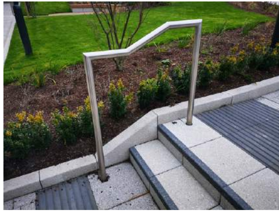
Stainless Steel Handrails
