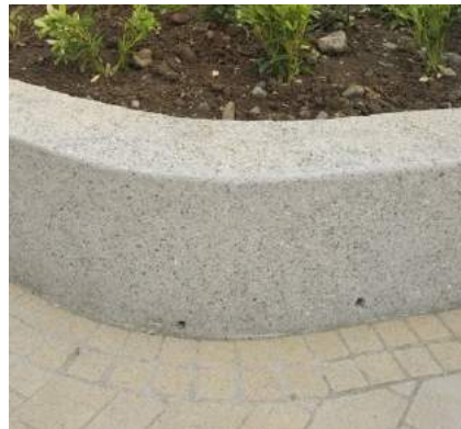
Exposed Aggregate Wall
