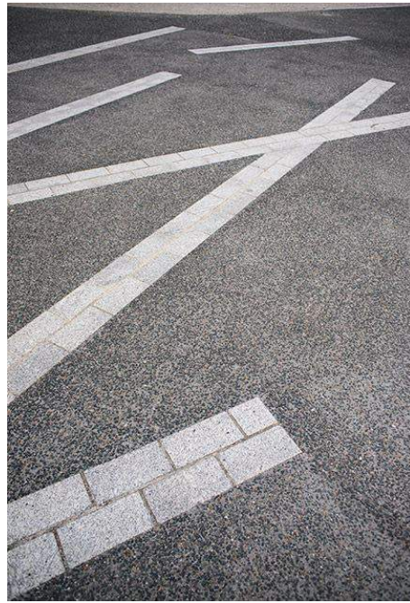
Exposed Aggregate Path in Local Park with PC concrete block bands
